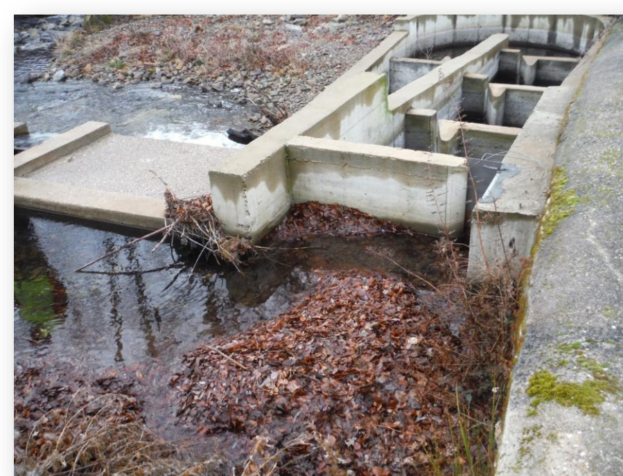
Figure 5. Example of an obstruction at the entrance of a fish pass, as result of a poor maintenance.
